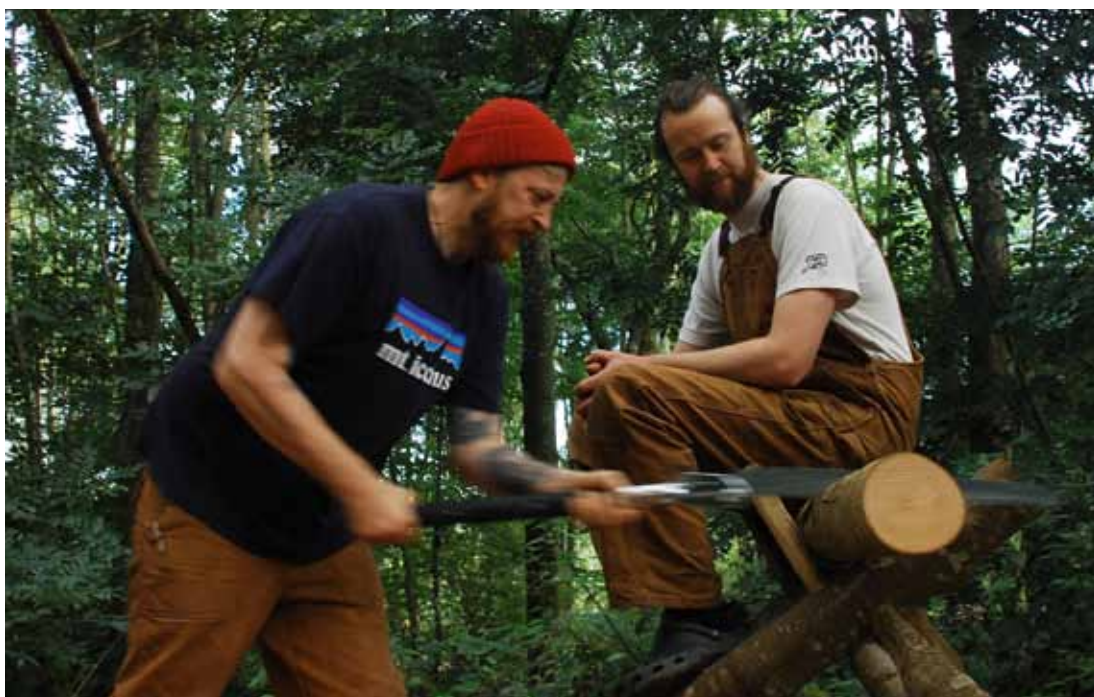
Will supervises the framing work
